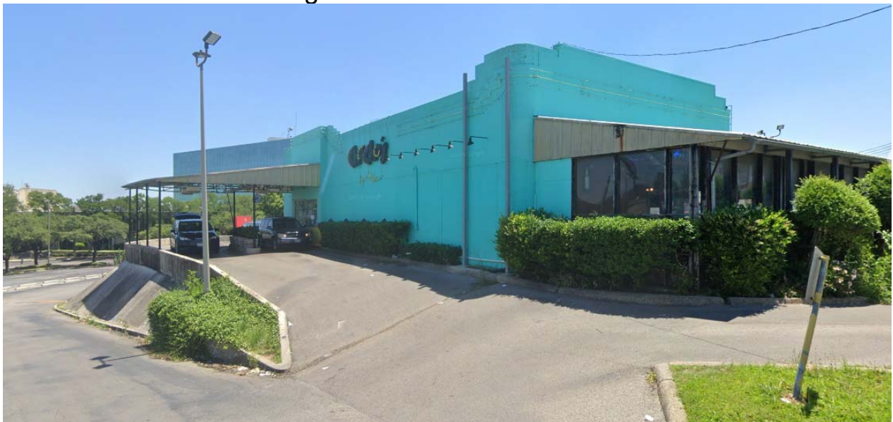
Drive Thru Side of Building
